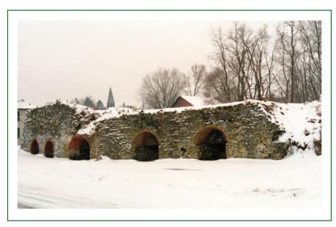
bottom, and the fire gradually spread upwards through the charge. When burnt through, the lime was cooled and raked out through the base.
